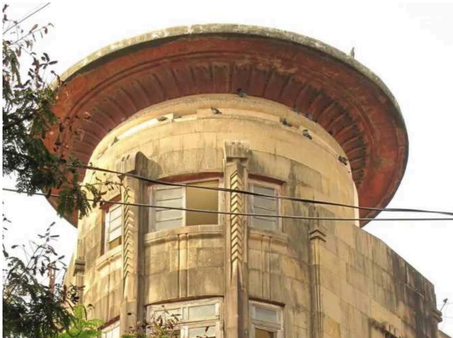
PNB house. Courtesy of Art Deco Mumbai Trust
