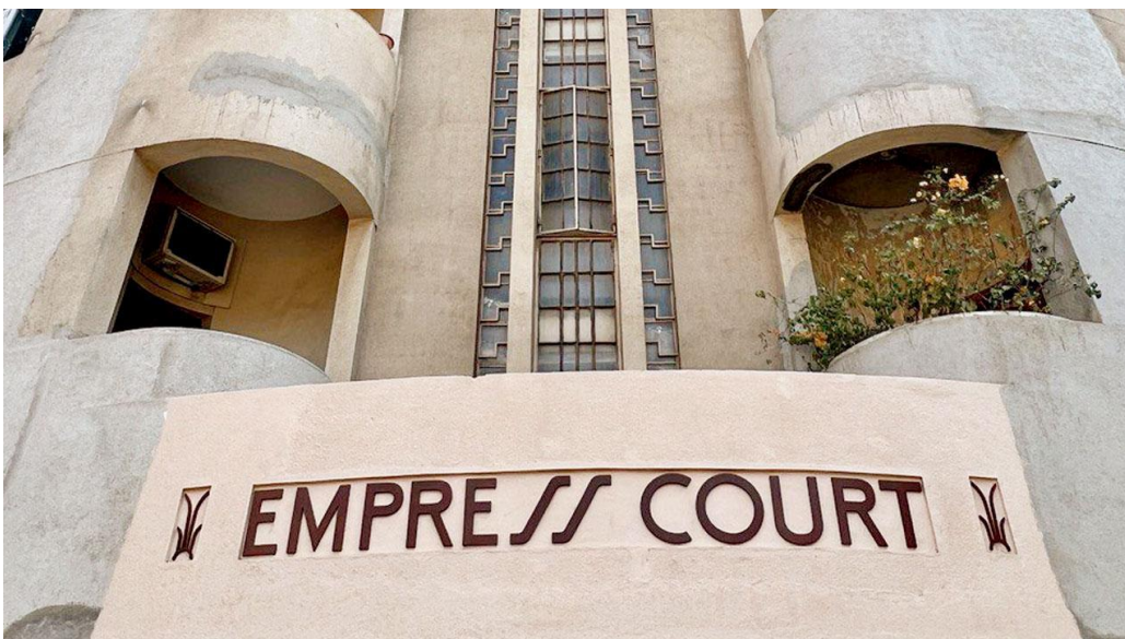
The new Empress Court lettering that is inspired from the original one, is made of metal. Pics courtesy/Art Deco Mumbai
