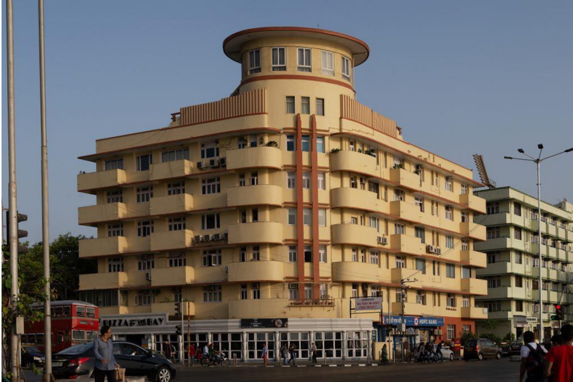
The Soona Mahal at Marine Drive
